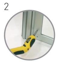
Assemble vertical profiles to the curved profile ensuring that the graphic fixing strip is adjacent to the post and facing forward (convex side).
